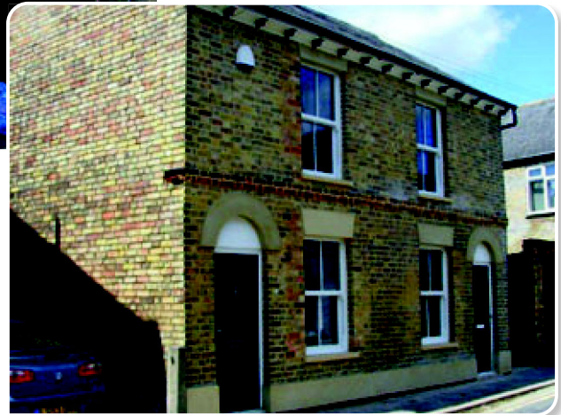
23/24 Great Northern Street, (After)
